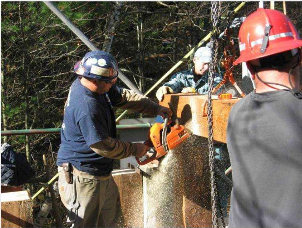
The contractor custom manufactured these blue service gains and attached them to the downstream side of the dam. They hold the logs in place that hold back the water while the olds logs are being removed and replaced.
