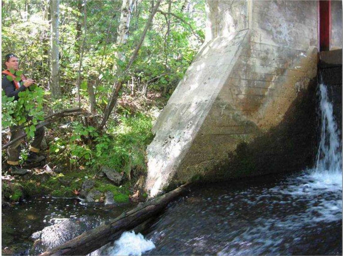
The contractor devised a scheme to place logs on the downstream side of the dam to temporarily block the flow. Without drive-up access, all materials were brought in by boat from a nearby marina. The 5 metre long fir logs do float but out of the water they weigh 200 kg each.
