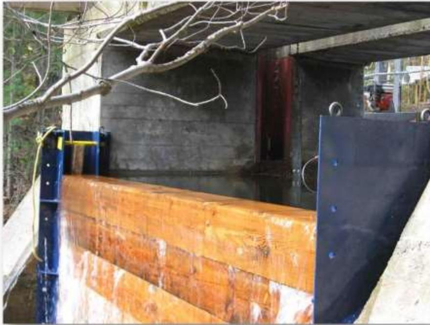
After the old logs were removed some debris in front of the dam was removed to make sure none of it would get stuck underneath the new bottom log or between the new logs. The new logs were then lowered down into place. This picture also shows one of the black jacks, beside the pail, that was to be used to jack the new logs down, pressing them into place and sealing any gaps between the logs to prevent water leakage.
