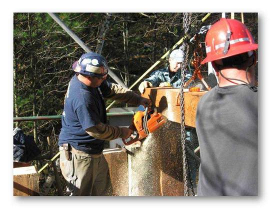
The contractor custom manufactured these blue service gains and attached them to the downstream side of the dam. They hold the logs in place that hold back the water while the olds logs are being removed and replaced.
