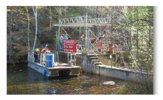
The temporary overhead gantry cranes were used to hoist the logs up from the water, move them from one side of the dam to the other and into position. Below, the temporary logs are being cut to the correct length to fit into the service gains, before being lowered into position.
