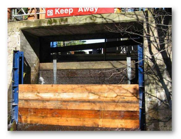
Using the flat pieces of steel on the old logs the contractor lifted them up a little, using a chain hoist. This allowed water to pass underneath the bottom log, flushing out the sill, and filling the space between the two sets of logs with water. The old logs began to float and a diver was used to unbolt them from one another so they could be lifted out separately.
