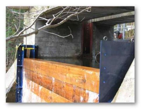
After the old logs were removed some debris in front of the dam was removed to make sure none of it wold get stuck underneath the new bottom log or between the new logs. The new logs were then lowered down into place. This picture also shows one of the black jacks, beside the pail, that was to be used to jack the new logs down, pressing them into place and sealing any gaps between the logs to prevent water leakage.
