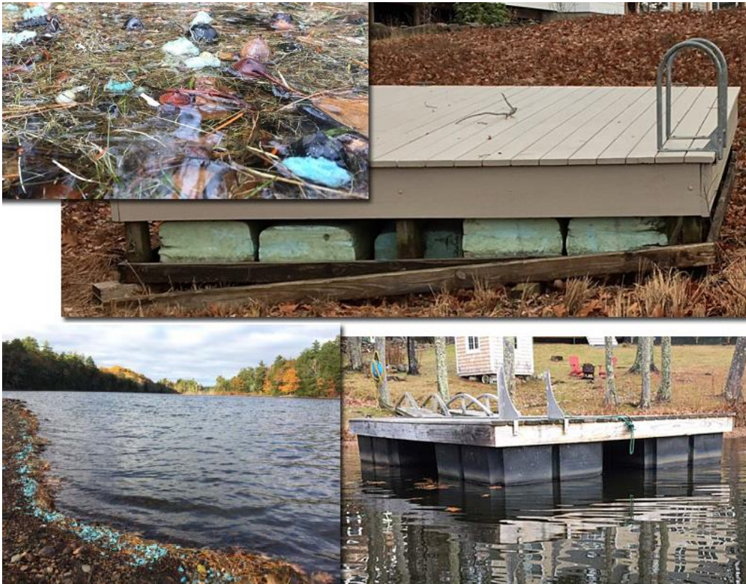
Debris top and bottom left. Dock with Polystyrene top right. Better alternative bottom right.
